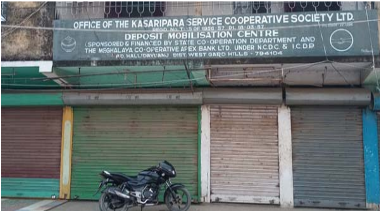
Office Building/ Deposit Mobilization Centre
