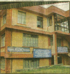
The complex of the Meghalaya Housing Financing Cooperative Society Ltd
